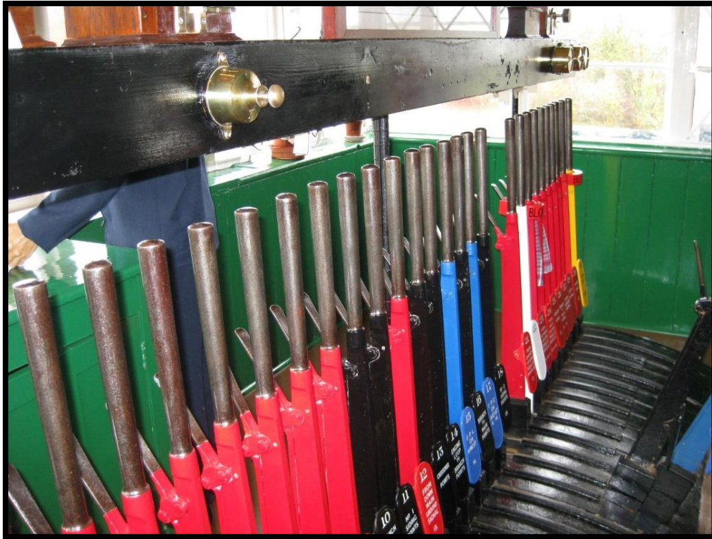
Interior of the restored box showing the point and signal levers.
