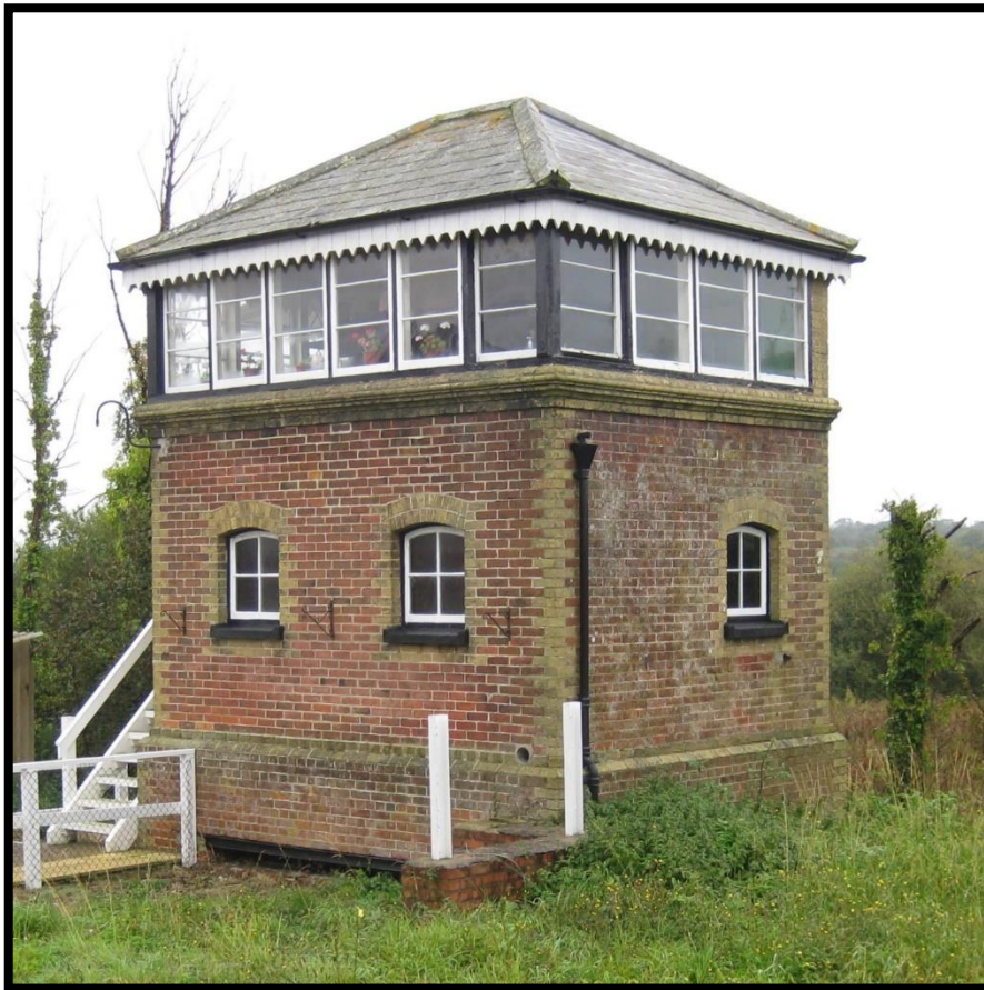
The Brading Signal Box was built in 1882 and contains the original mechanisms.
