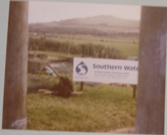
Old sewer beds renewed '09
