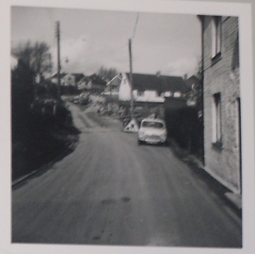
WEST STREET BEFORE 6-30 RING WIDENING cont'd. from page 47
