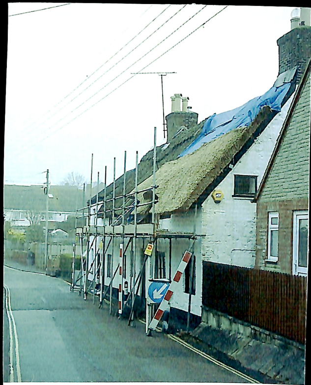
Renewal of thatching on Tortola Cottage MARCH 2002
