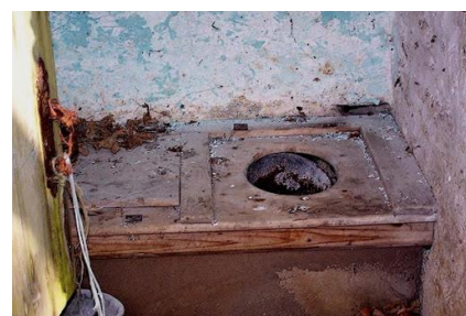
An example of a Victorian privy or toilet
